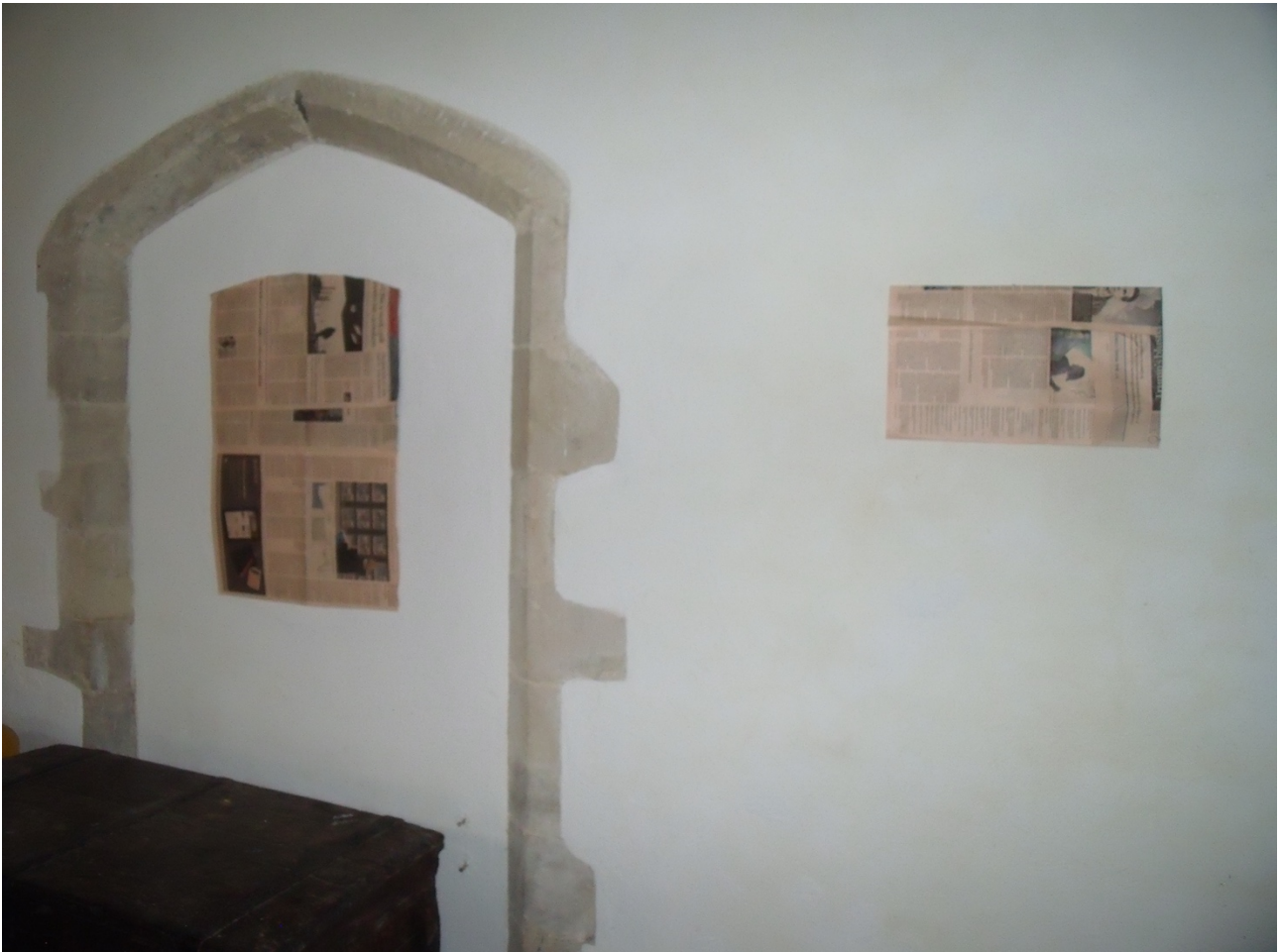
North Aisle – East portion – to be (paper mock-up)
